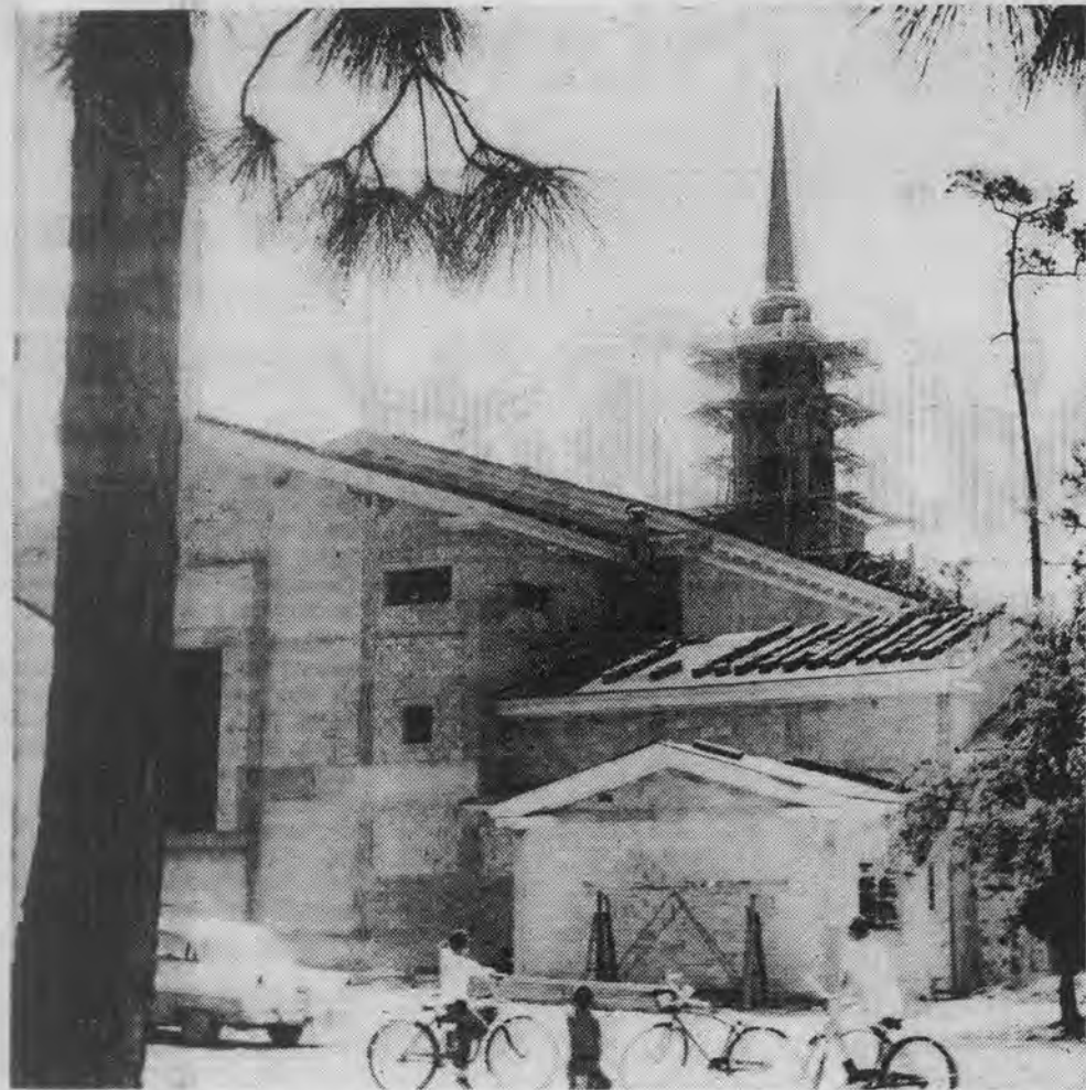
BOYS WATCH WORK ON GRANADA PRESBYTERIAN SANCTUARY
