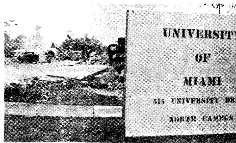
University Sign Remains ... as crew cleans up rubble
